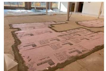
The fire-treated plywood was left in place. High strength, but also lightweight, extruded polystyrene insulation panels were placed in the low spots across the subfloor.
