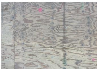
Fire-treated plywood covered the space, providing a surface which met code requirements, but one with bonding issues for subfloor materials.
