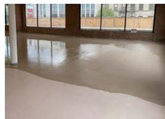
Schönox AP Rapid Plus's hybrid active-dry technology allowed the leveler to dry independently of job site temperature and humidity conditions.
